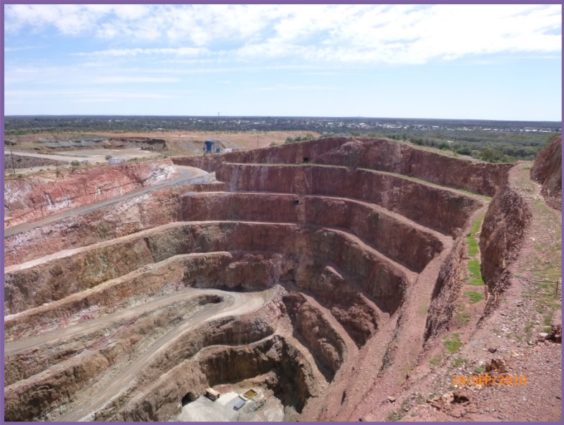
open cut mining the Cobar way
