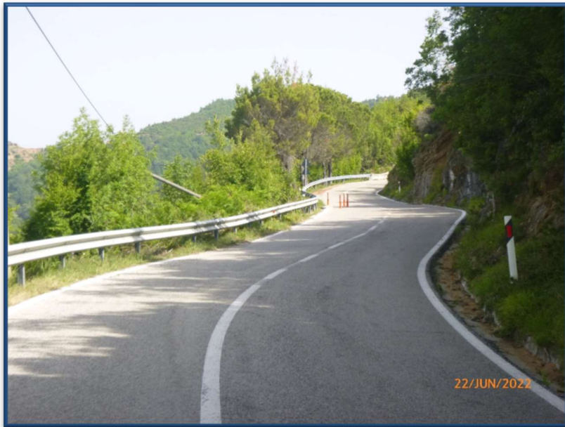
must be a significant pot-hole to warrant this attention
