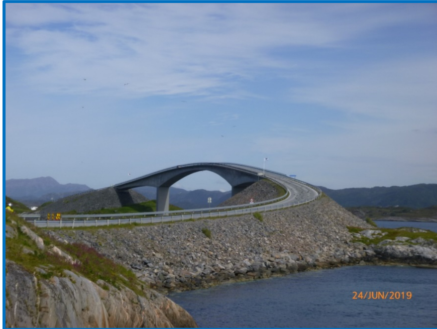
Atlantic Road Bridge
