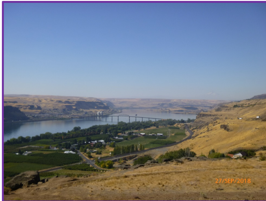
Sam Hill Memorial Bridge and the Columbia River, viewed from Stonehenge Memorial
