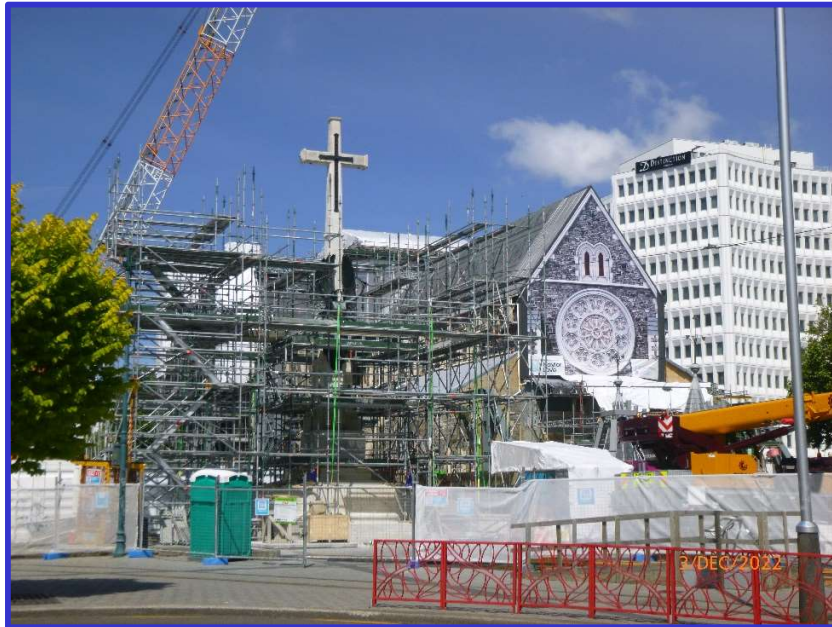
Christchurch Cathedral reconstruction works
